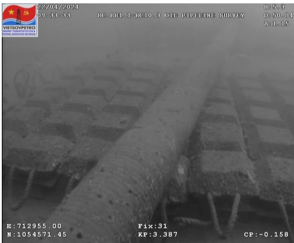
Figure 43: Concrete mattress #3
