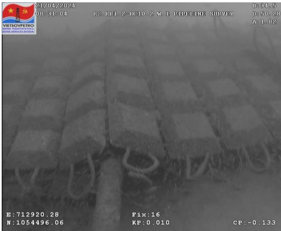
Figure 45: Concrete mattress #2
