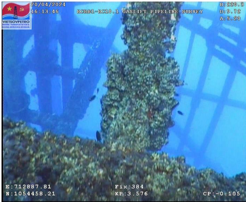
Figure 18: Riser clamp at EL -10m
