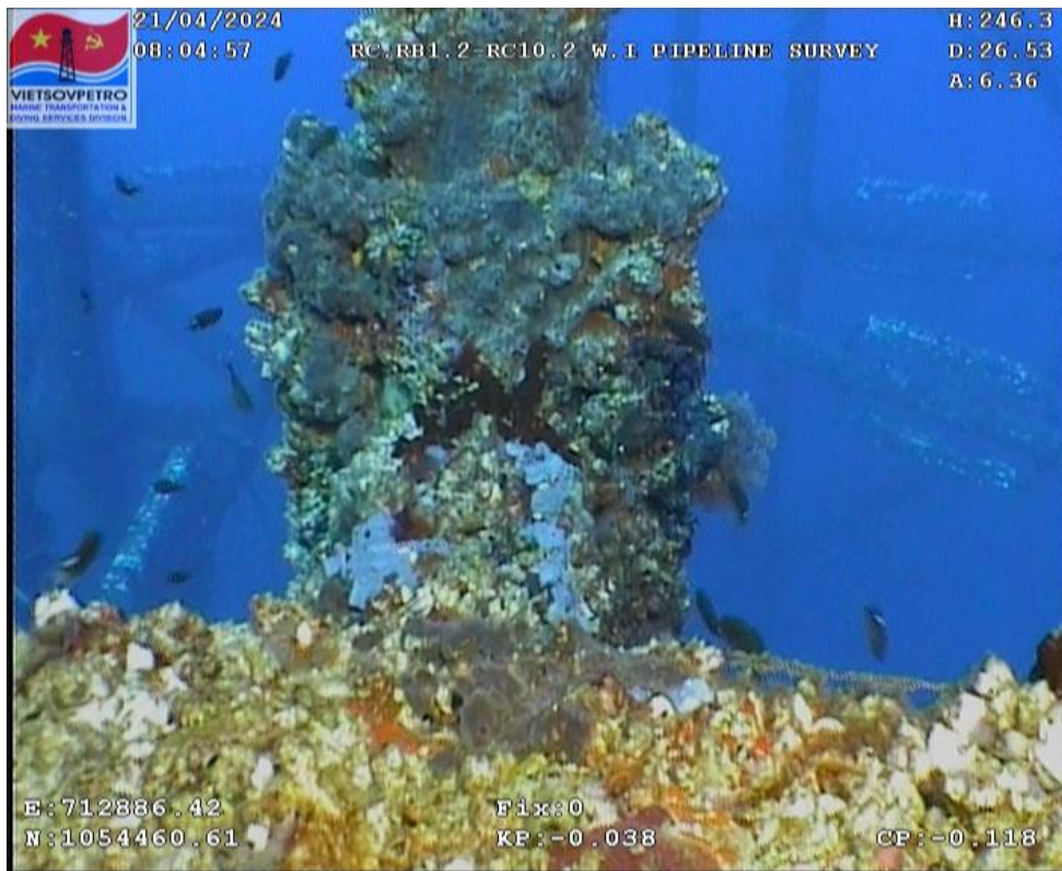
Figure 8: Riser clamp at EL -27m
