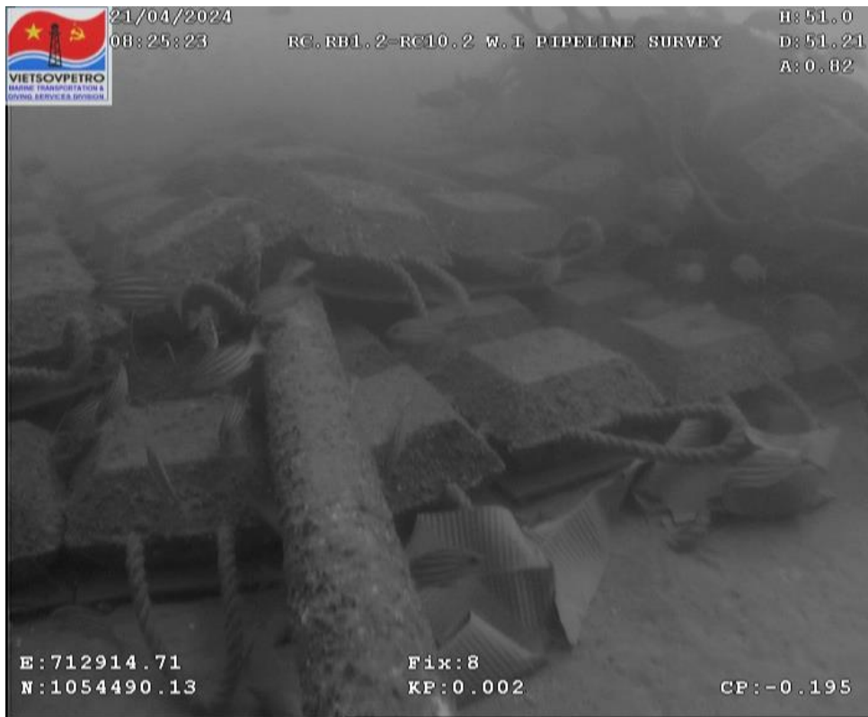
Figure 44: Concrete mattress #1
