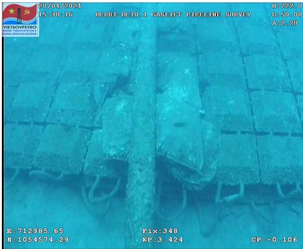
Figure 52: Concrete mattress #6
