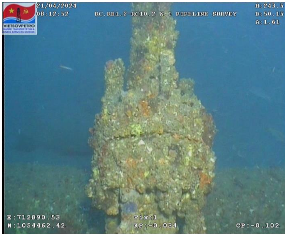
Figure 40: Tie-in point at Fix.1
