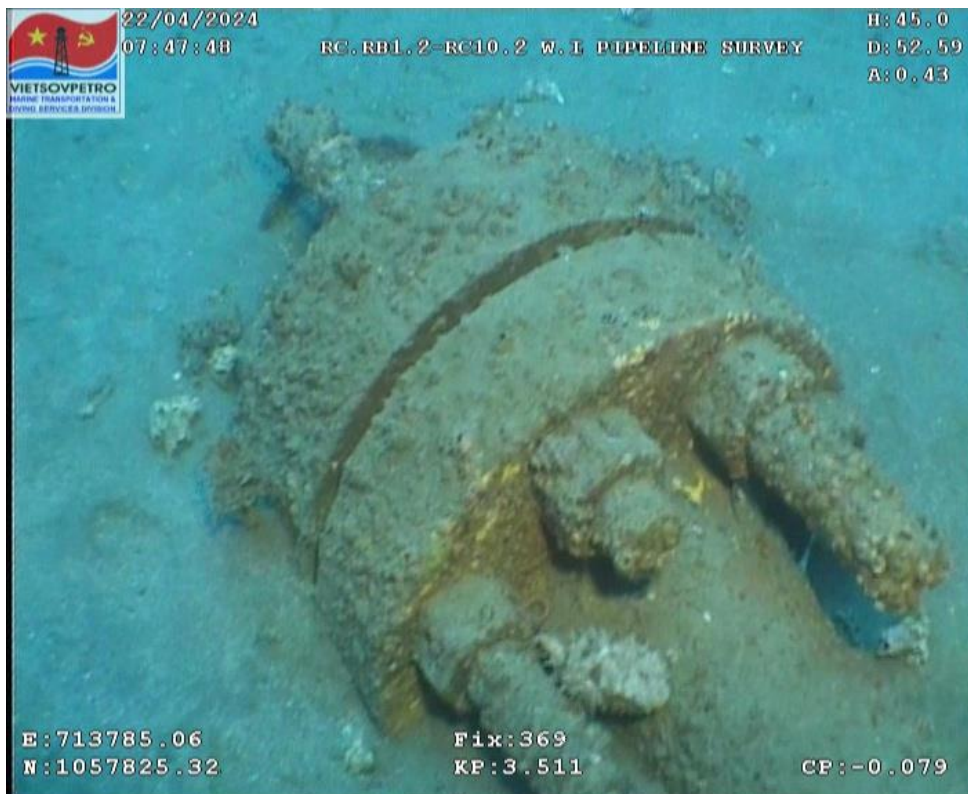
Figure 42: Tie-in point at Fix.369
