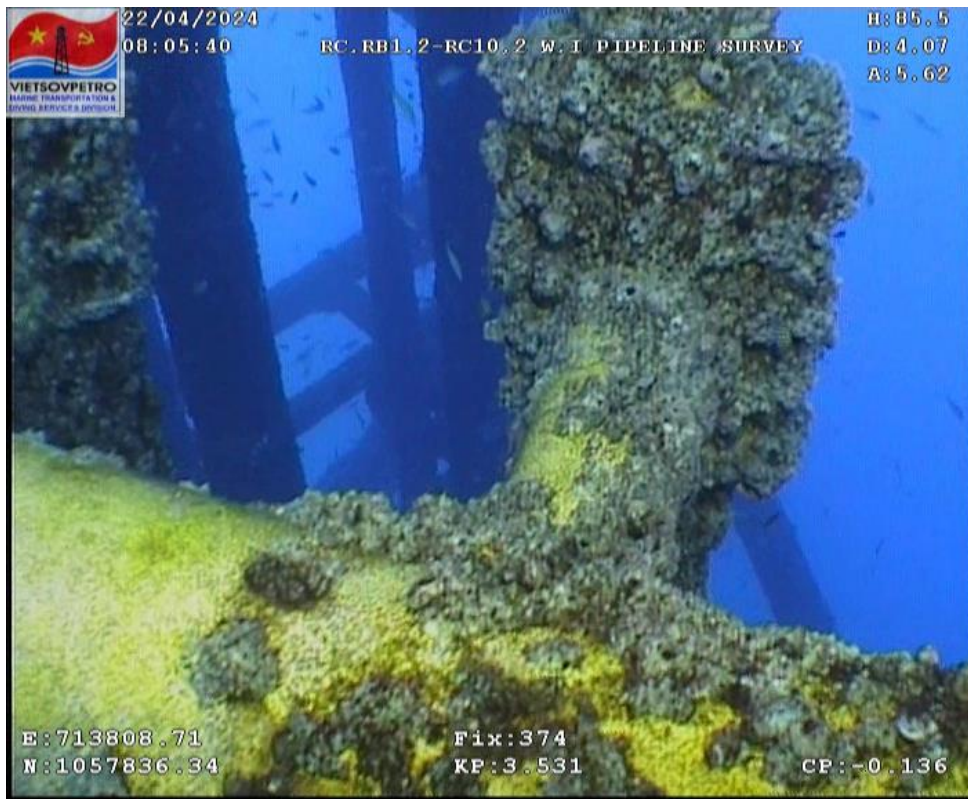
Figure 15: Riser clamp at EL -5m
