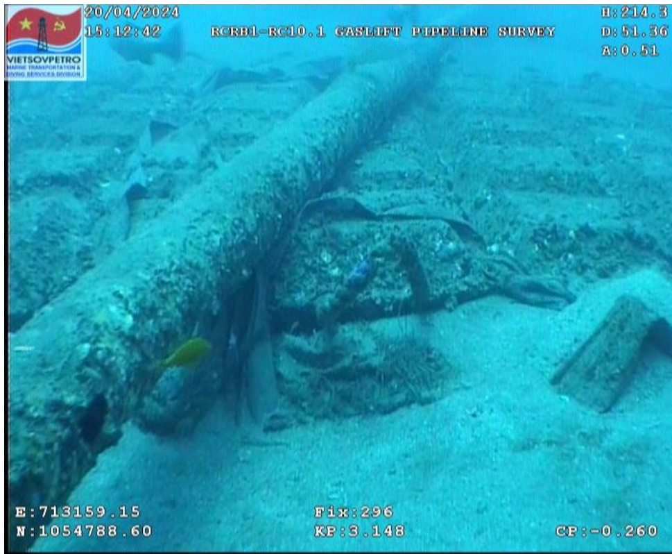
Figure 47: Concrete mattress #1
