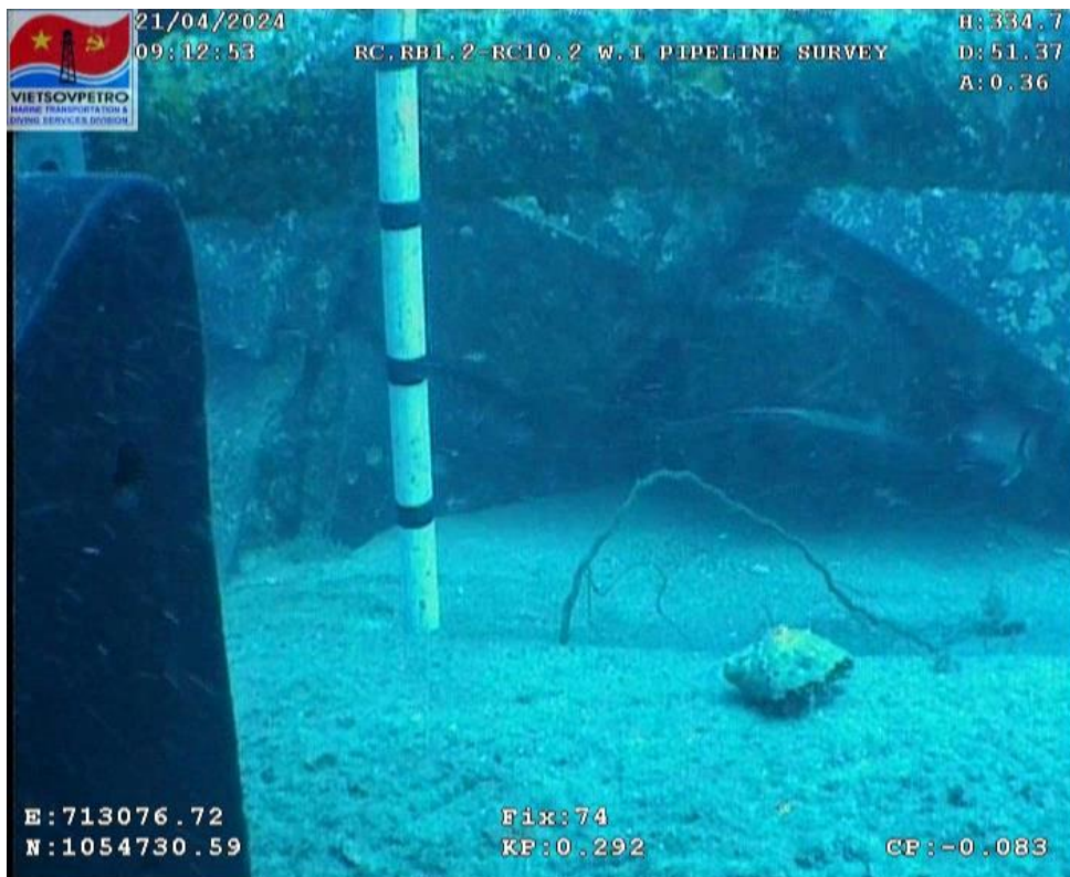
Figure 28: Gap between 02 pipelines at Fix.74
