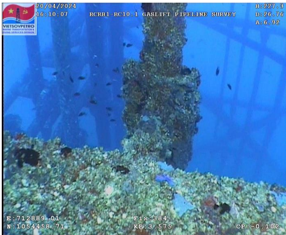
Figure 21: Riser clamp at EL -28m
