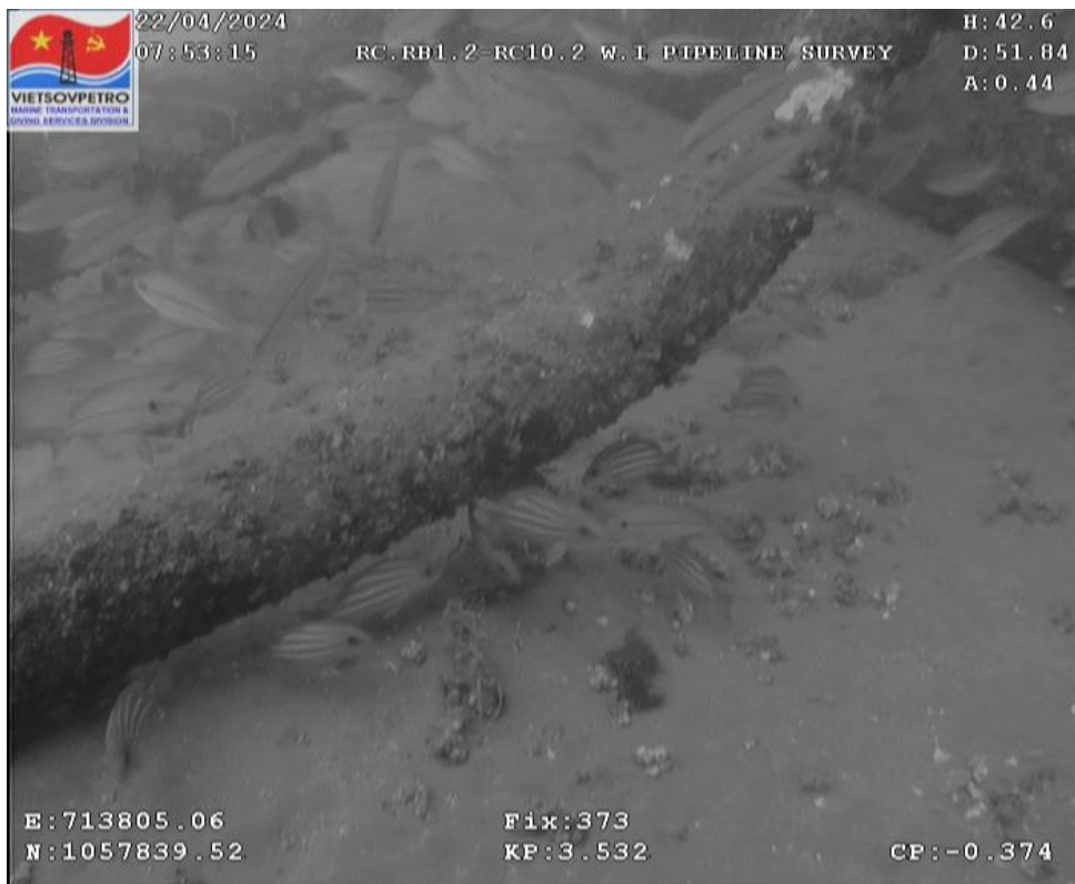
Figure 24: Riser elbow
