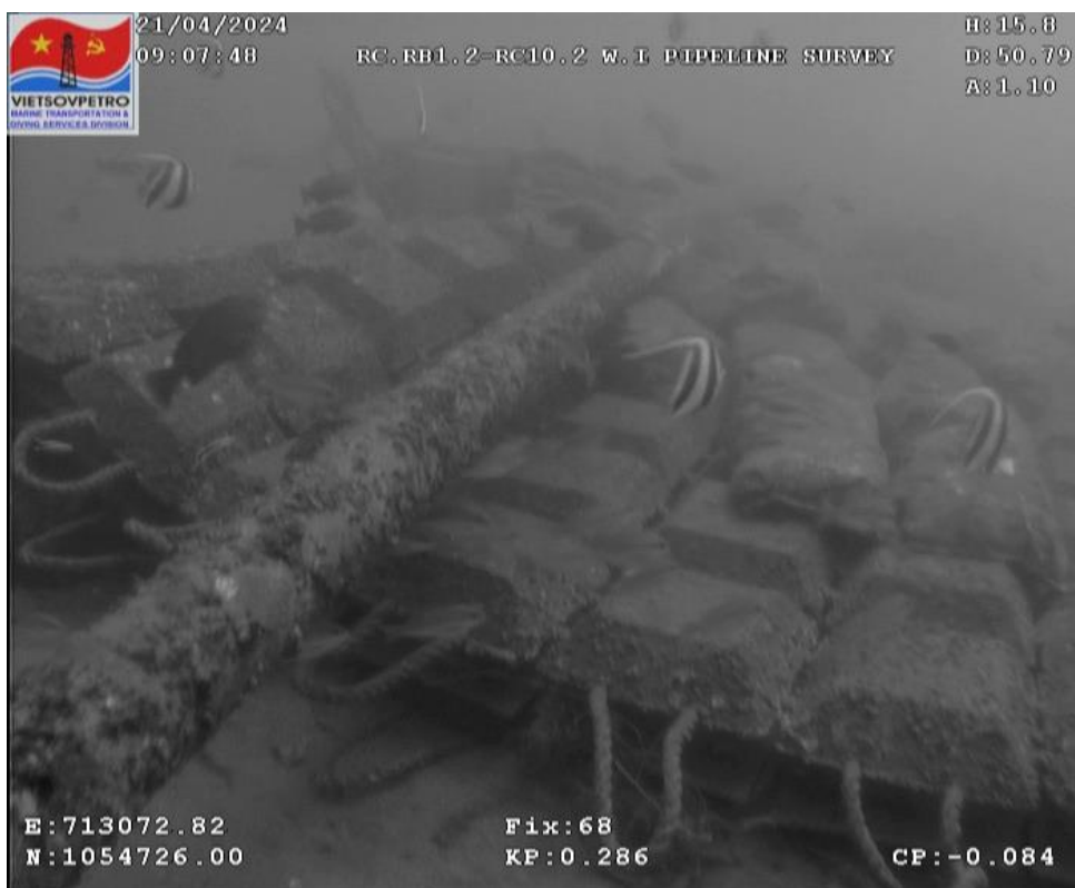
Figure 48: Concrete mattress #5
