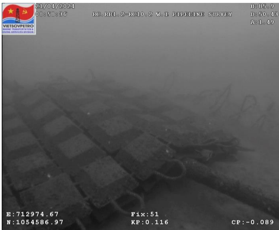
Figure 47: Concrete mattress #4
