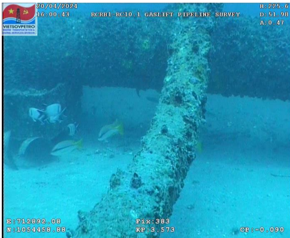
Figure 25: Riser elbow
