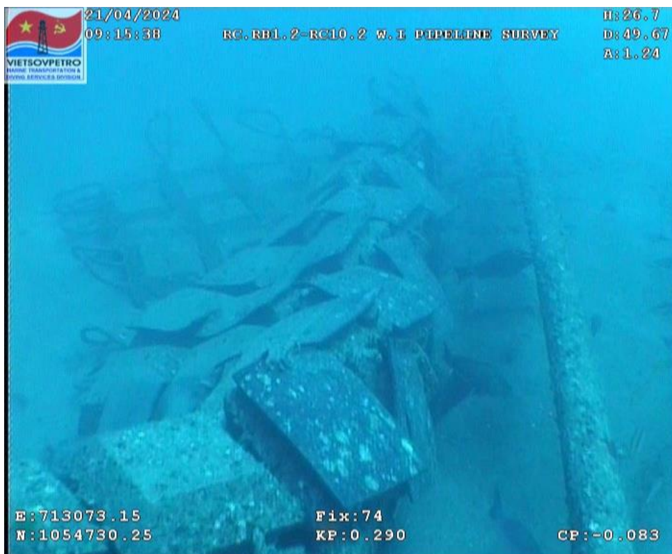
Figure 53: Concrete mattress making a roll (#9)
