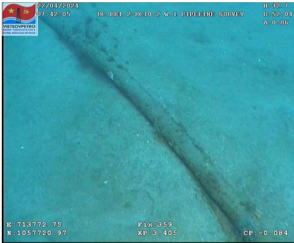
Figure 29: Crossing under power cable without support at Fix.359
