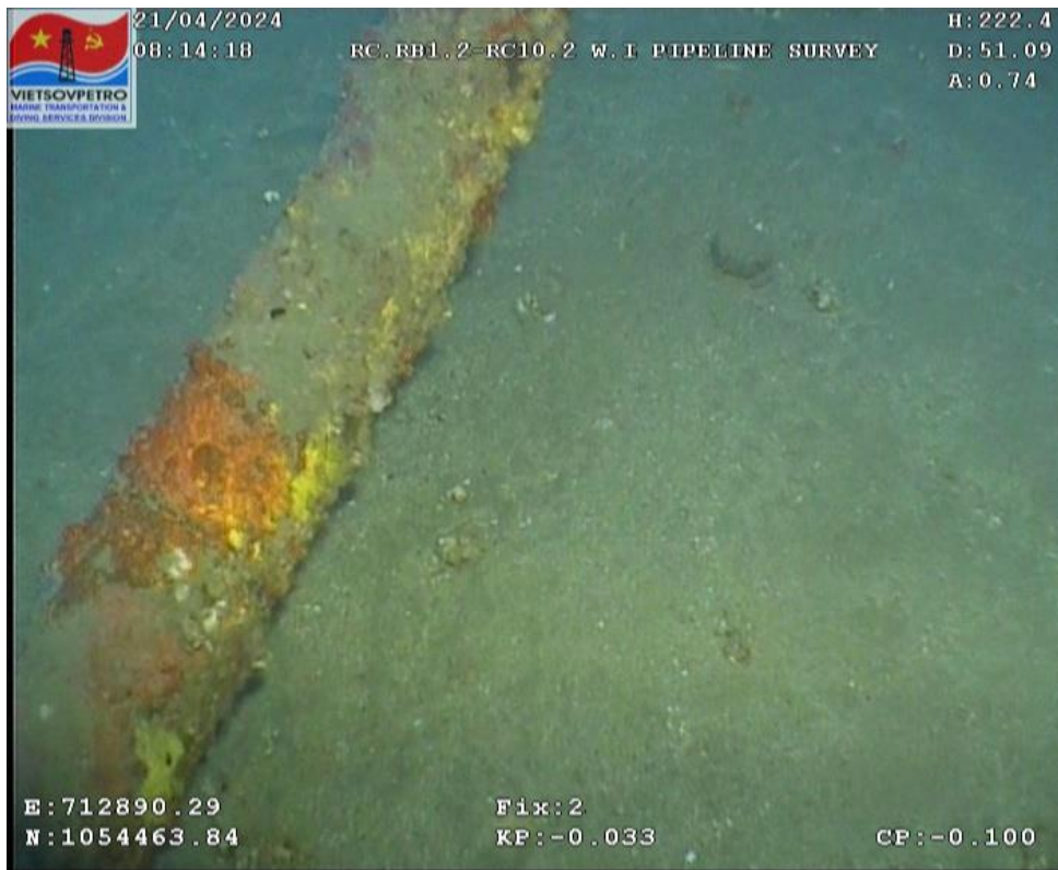
Figure 12: Riser elbow
