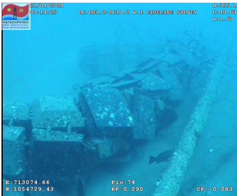
Figure 52: Concrete mattress making a roll (#9)
