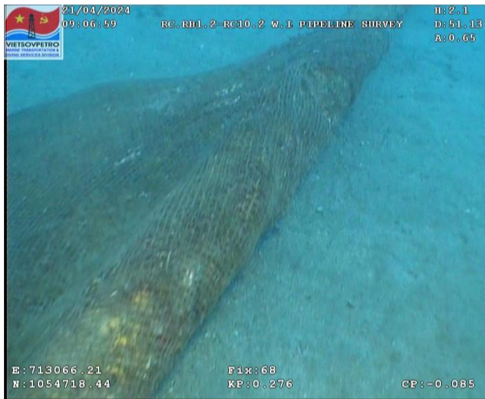
Figure 26: Debris soft netting at Fix .68
