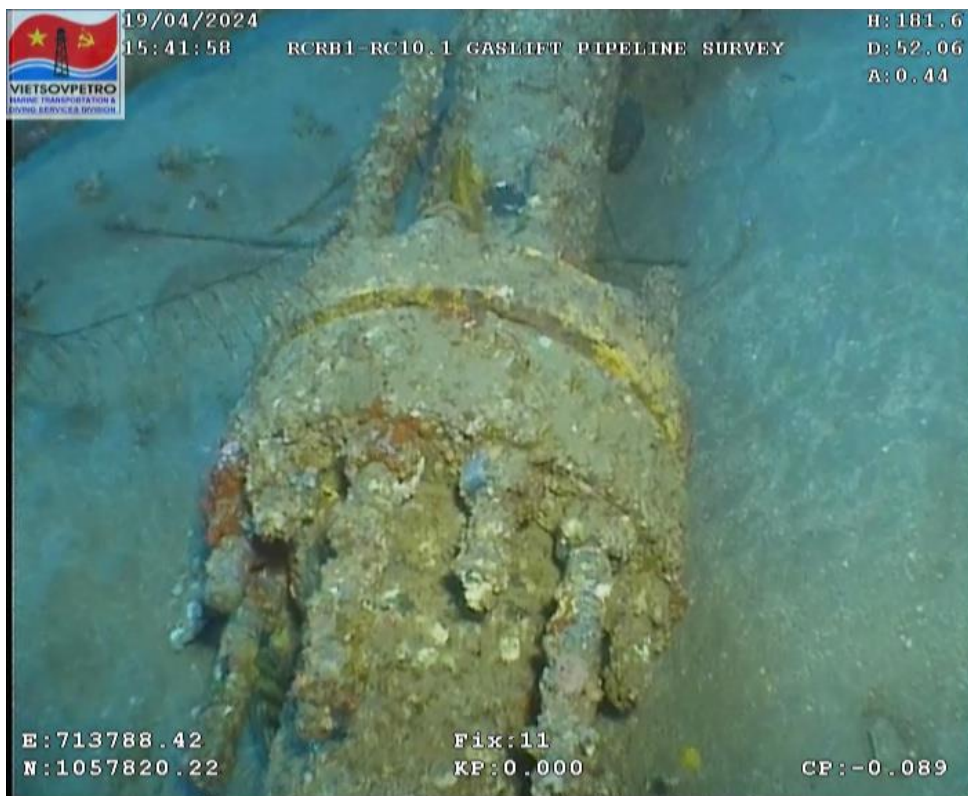
Figure 44: Tie-in point at Fix.11
