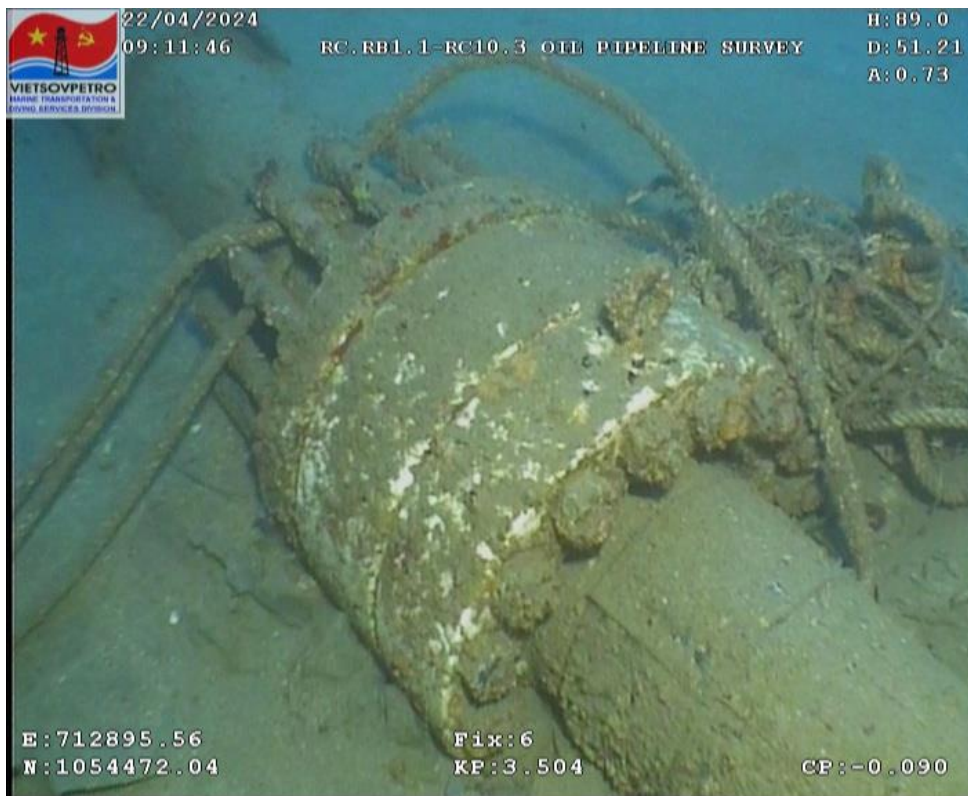
Figure 38: Tie-in point at Fix.6
