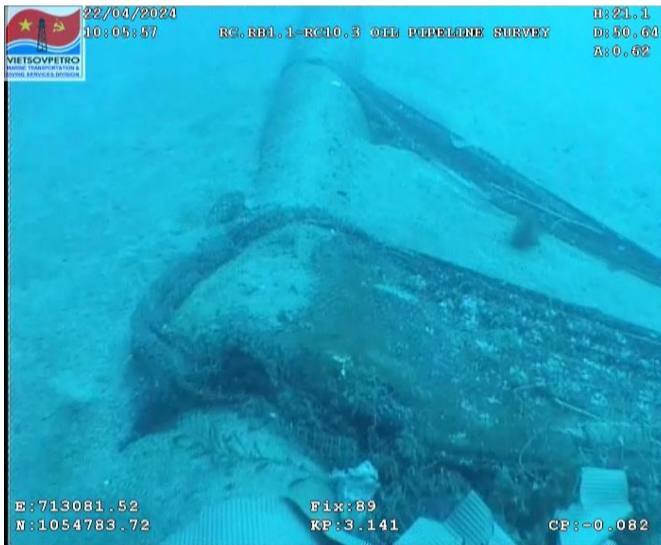
Figure 24: Debris soft netting at Fix .89
