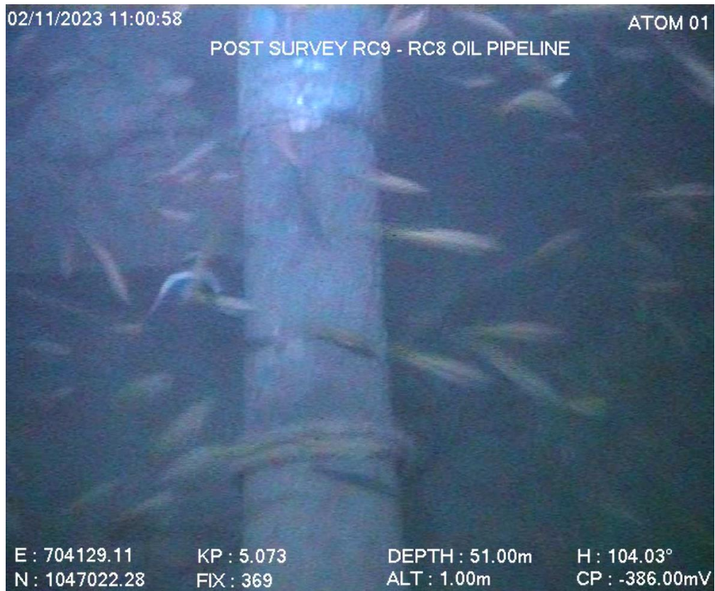
Figure 11: RC8 riser elbow condition
