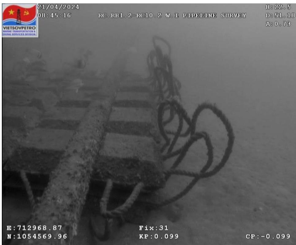
Figure 46: Concrete mattress #3
