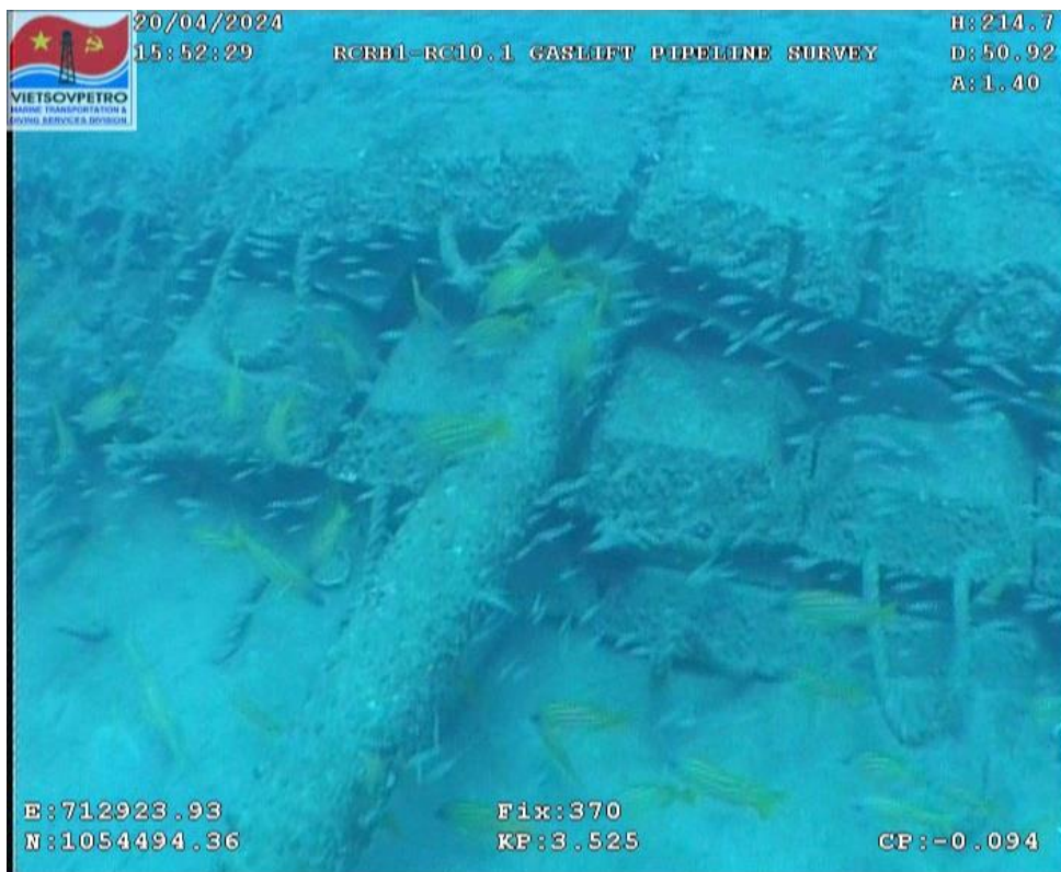
Figure 54: Concrete mattress #8
