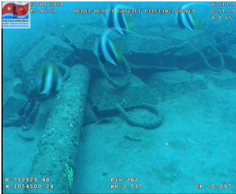
Figure 53: Concrete mattress #7
