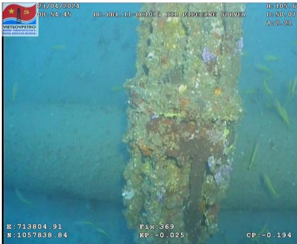
Figure 40: Tie-in point at Fix.369
