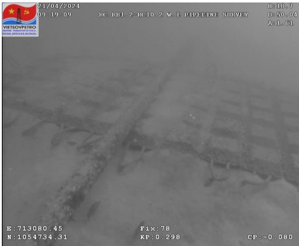
Figure 51: Concrete mattress #8
