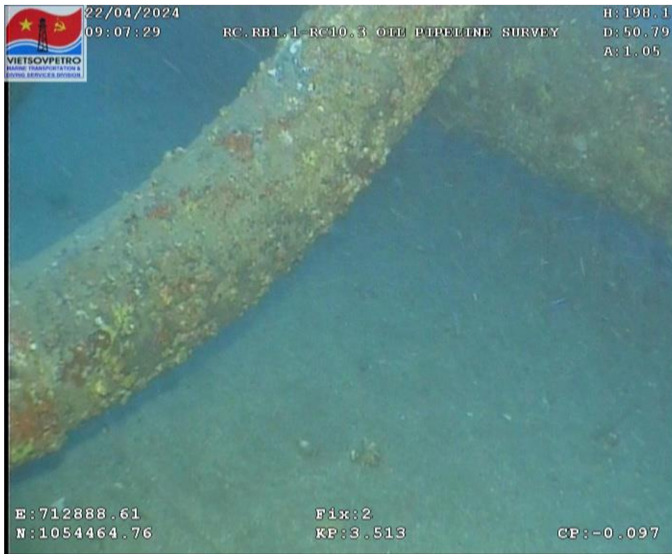
Figure 10: Riser elbow
