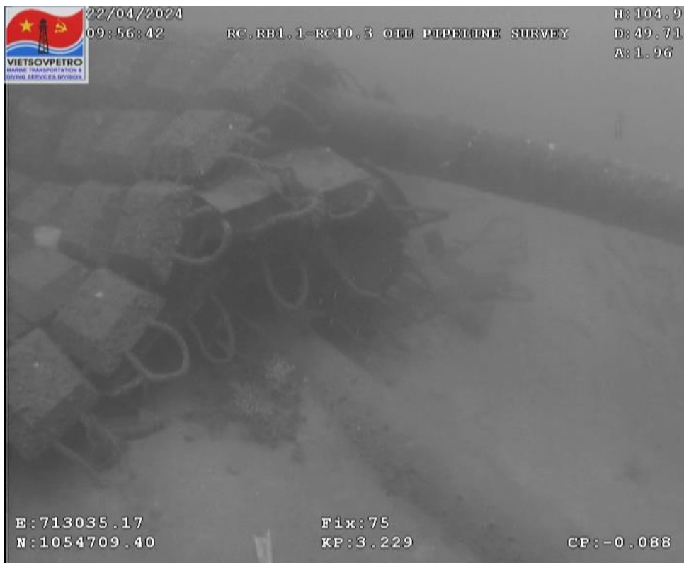
Figure 48: Concrete mattress #8
