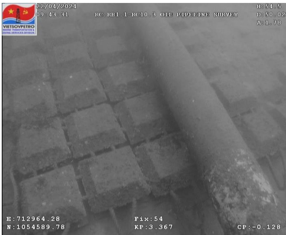
Figure 46: Concrete mattress #6
