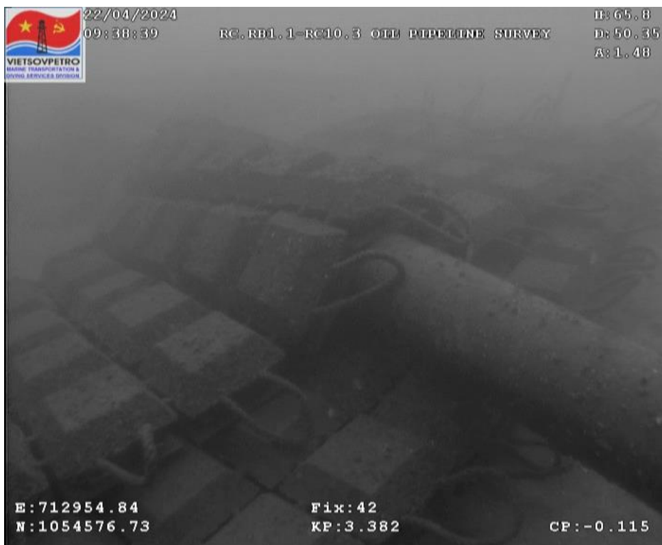
Figure 44: Concrete mattress #4
