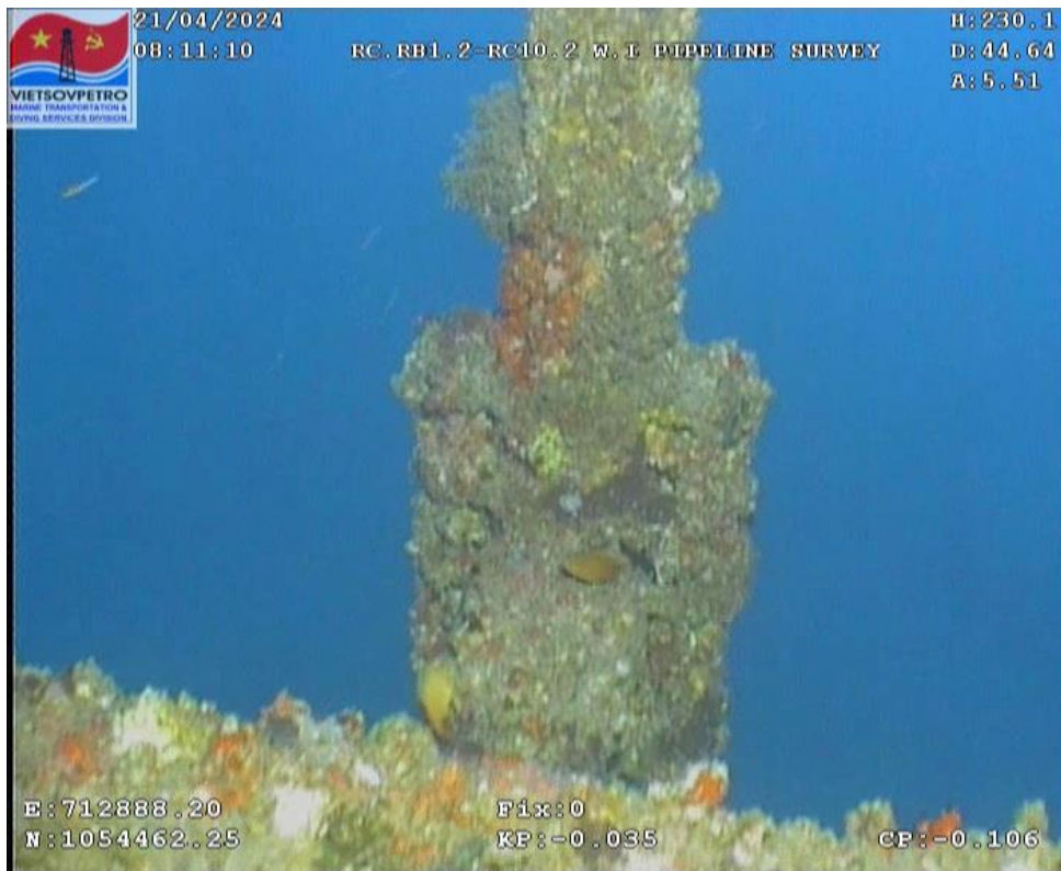
Figure 11: Riser clamp at EL -46m
