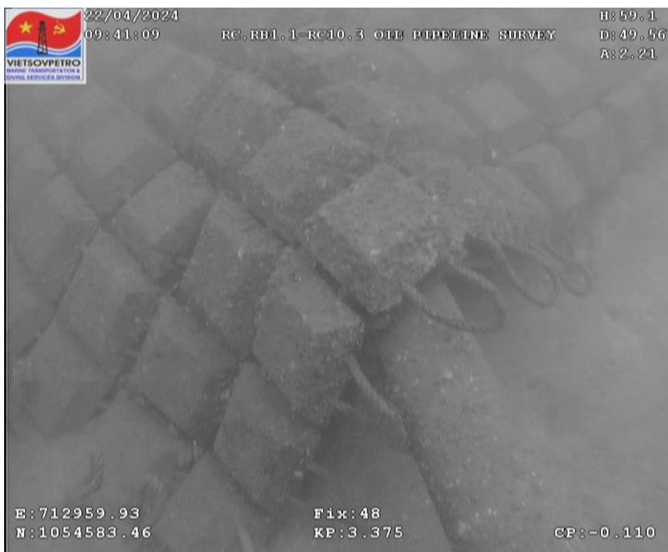
Figure 45: Concrete mattress #5
