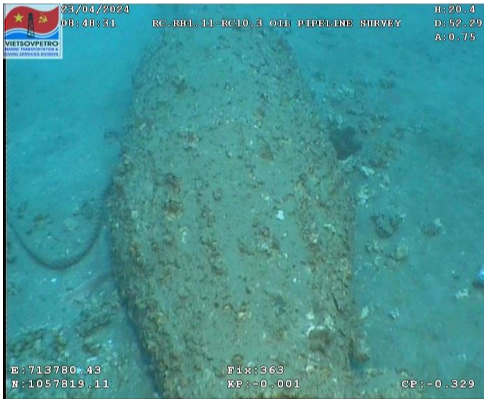
Figure 39: Tie-in point at Fix.363
