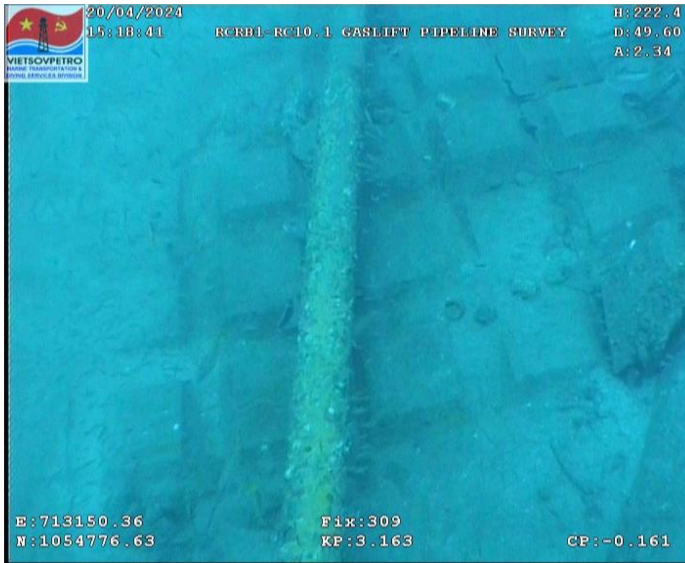
Figure 49: Concrete mattress #3
