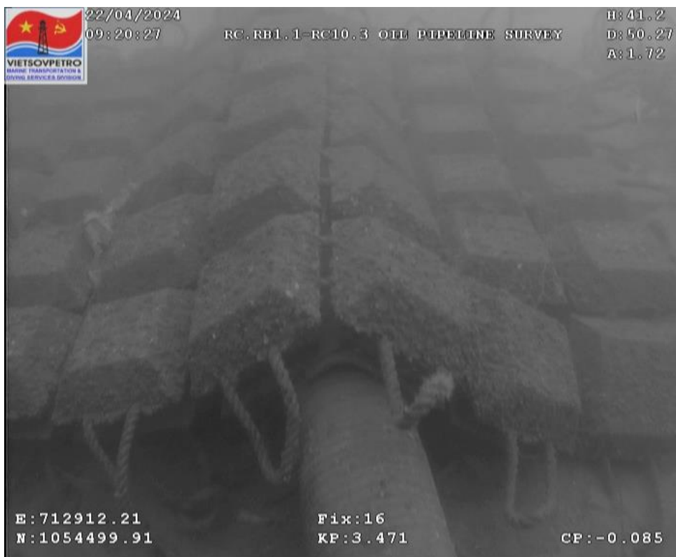
Figure 42: Concrete mattress #2
