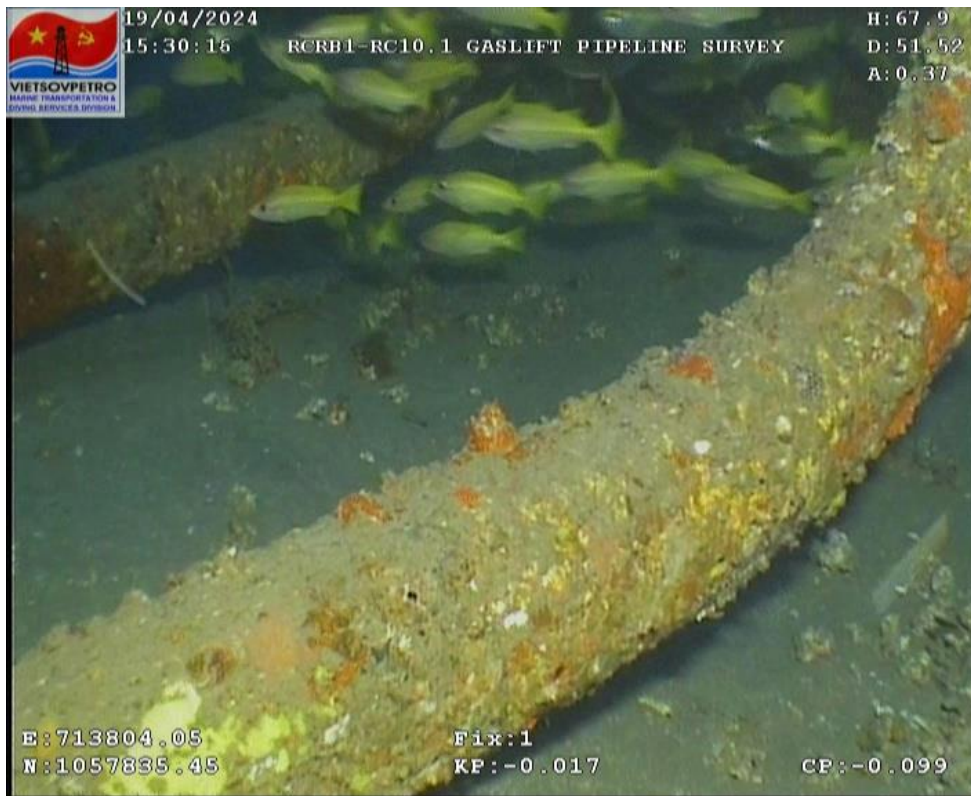
Figure 13: Riser elbow
