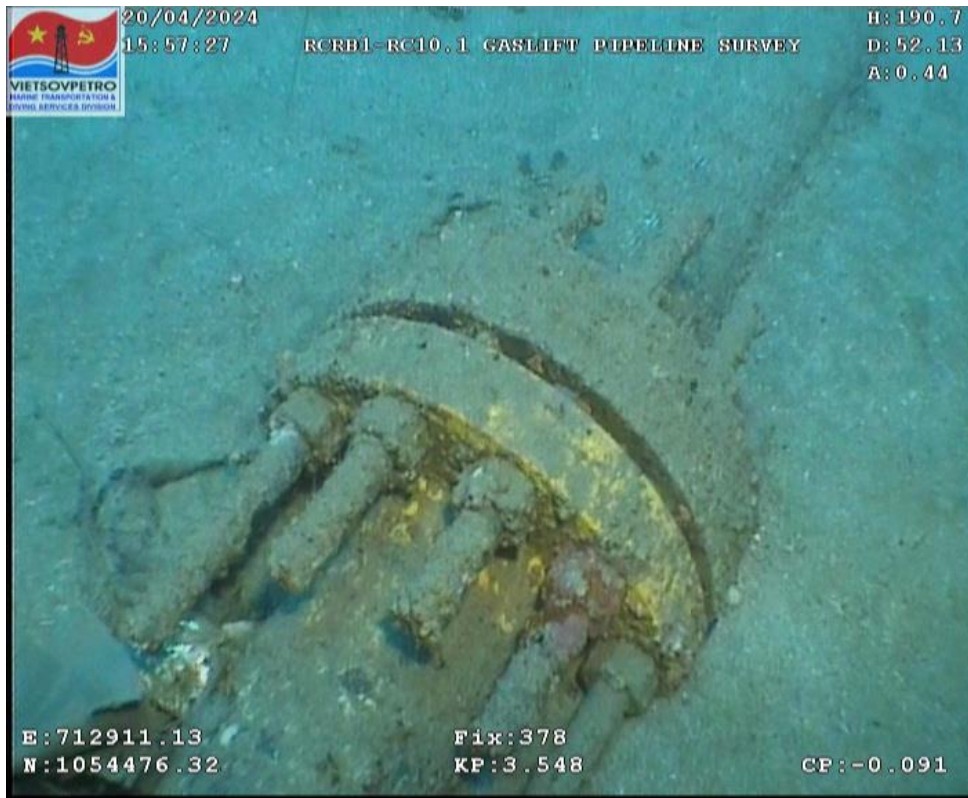
Figure 45: Tie-in point at Fix.378
