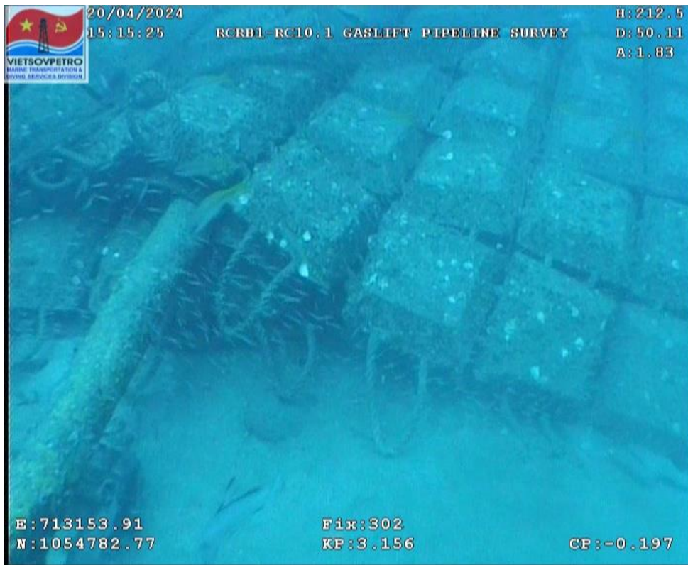
Figure 48: Concrete mattress #2
