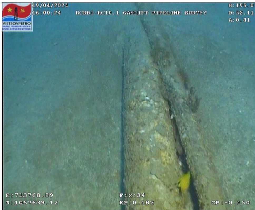
Figure 29: Crossing under power cable without support at Fix.34
