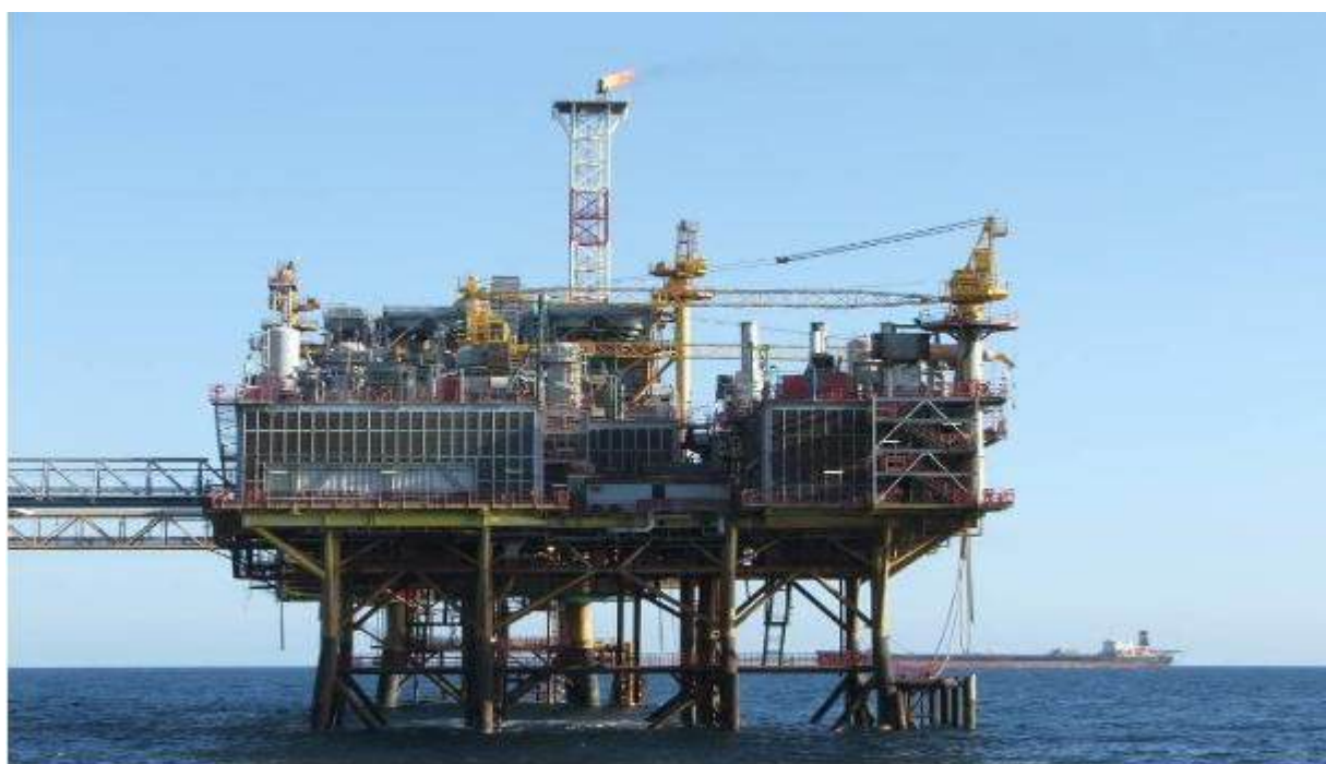
Fig. 1.1 – The WIP40000 overview
